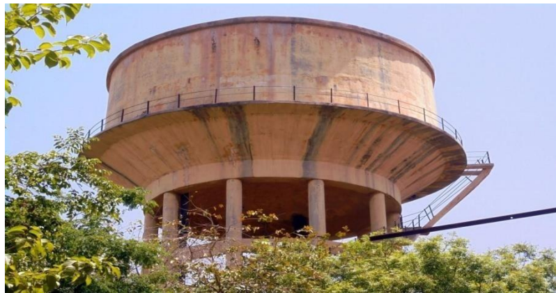
Fig1.6 Overhead Water Tank
